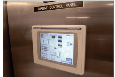
*The custom built Turbine Control Panel used Allen-Bradley SLC500 PLC and Panelview Plus HMI.*
