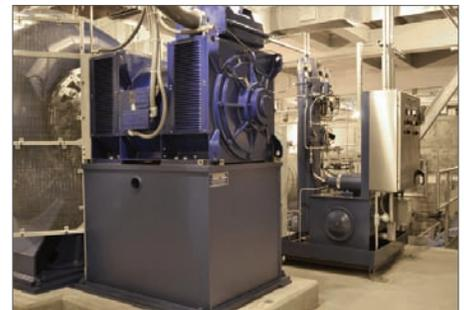
*The 200 kW, 480 VAC, 3PH, 60 Hz, 727 rpm induction generator was manufactured by Marelli Motori.*
