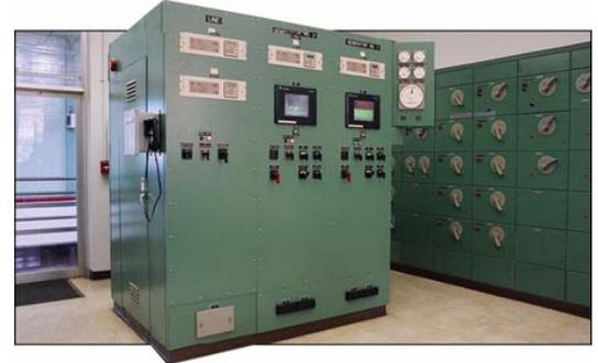
Sorensen Governor provided turbine rehabilitation, governor conversion and station automation for the MWRA facility to monitor and control the flow of water for the City of Boston.
