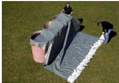
(8) Plastic membrane is positioned up to cylinders and fixed with a few sandbags, sealing the barrier.
