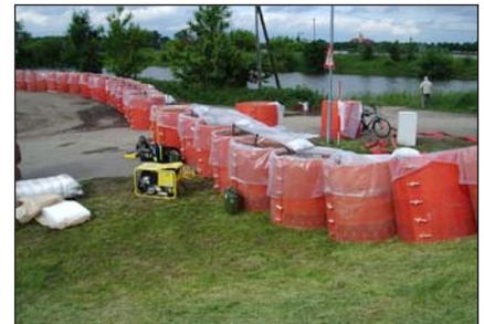
(9) The deployed cylinders provide a reliable flood defense that can be quickly dismantled after use.
