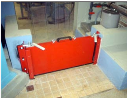
Manual containment barrier for pedestrian access.
