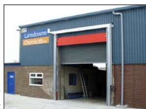
Automatic drop-down barrier.
