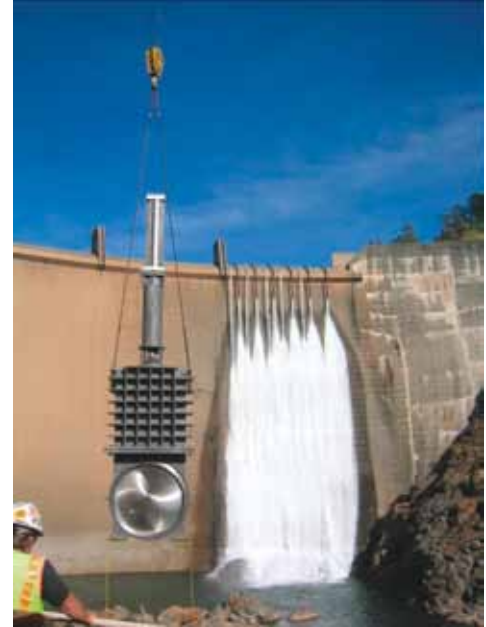
78" Hydro Guard Valve, 130 psi, CS with 304 SS Trim, For Fixed Cone Valve Isolation, Englebright Dam, California
