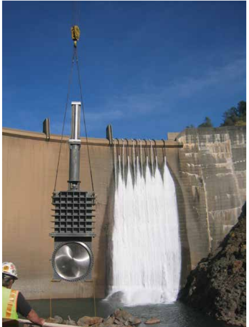
A 72" Hilton Bonneted Knife Gate Valve (130 psi rating) with 18" diameter hydraulic cylinder actuator is used for a guard valve for a fixed cone valve.
