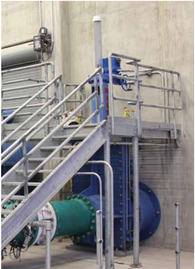
A 24" Jet Flow Gate (150 psi rating) with motor operator on a dam in Southern California.
