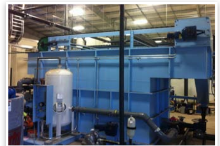
DAF Unit Using Conventional Recycle System.
