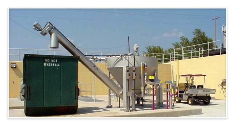
The Kusters Water ProTechtor<sup>™</sup> Grit Washer is known for its reliable operation and robust design. Separation efficiencies of the grit washer are much higher than conventional grit classifiers. All ProTechtor<sup>™</sup> products are US Manufactured at Kusters Water's ISO 9001:2008 certified facility.
