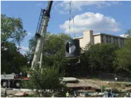
Offloading a Vortex Top Form.
