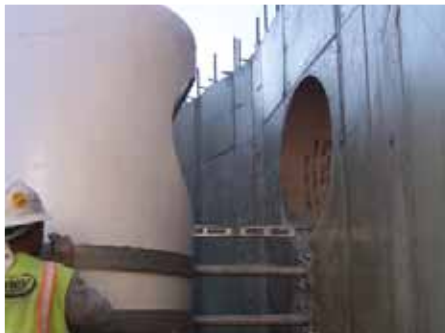
Strapping detail on Vortex unit, Buckeye, Arizona.
