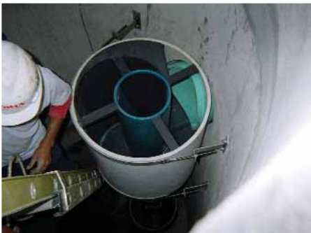
Vortex unit being strapped and adapted to inlet pipe.
