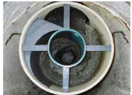
Vortex Flow Insert reducing H 2 S concentration levels, Camden County, New Jersey.
