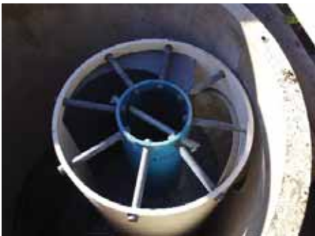
Vortex Top Form to be secured to structure, Alexandria.
