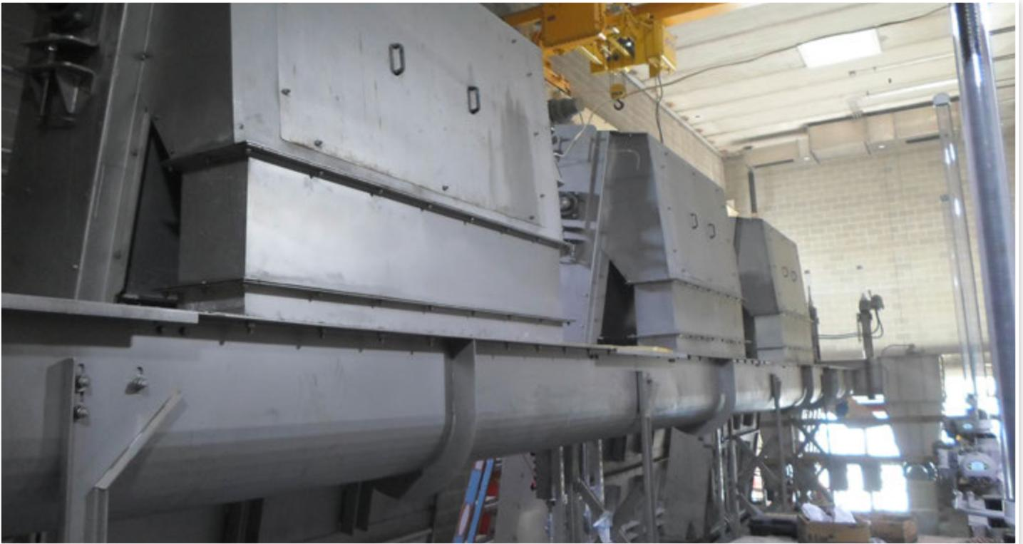
The Kusters Water ProTechtor™ Multi-Rake Bar Screen combines fine or coarse screening with high solids capture rates. Its robust construction and overload feature ensure reliable operation.
