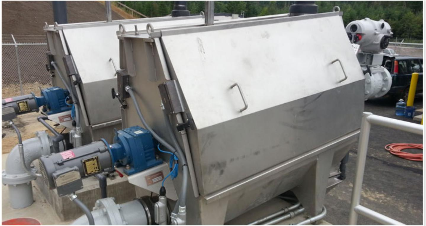
The highly efficient Internally Fed Drum Screen offers low water usage and low energy consumption, while maximizing screening efficiency.
